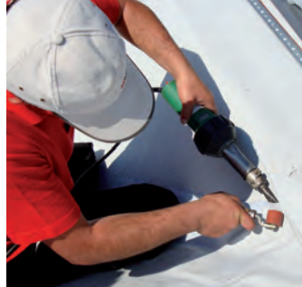
Welding a patch with the TRIAC PID on a building site.
