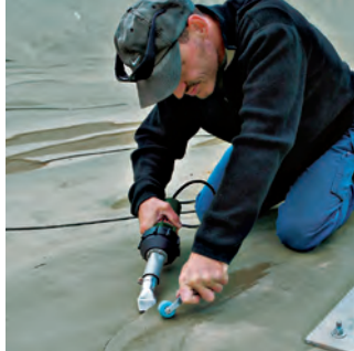
Welding of the connectors with TRIAC PID and push-fit wide slot nozzle.
